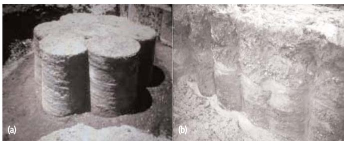
Fig 2. Examples of constructed columns using soil mixing augers: (a) overlapping configuration and (b) barrier wall configuration.
