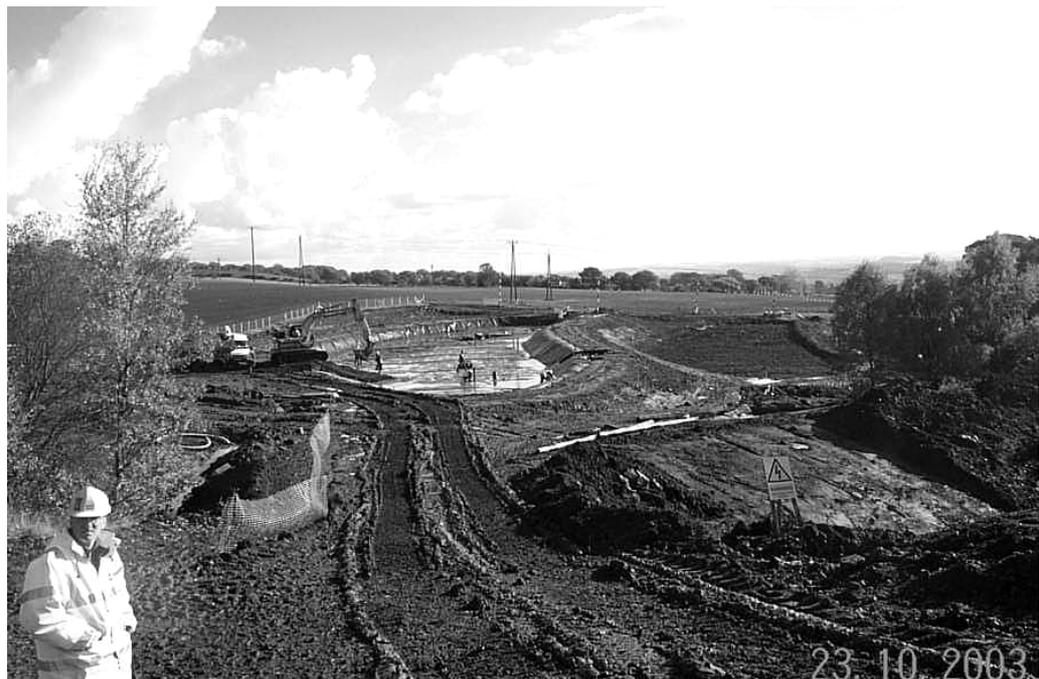
Figure 4.4: Earthworks for the full-scale treatment system at Bowden Close. In the background are the two RAPS lagoons. Only RAPS lagoon No 1 (to the left) has an artificial High Density Polyethylene (HDPE) liner.
