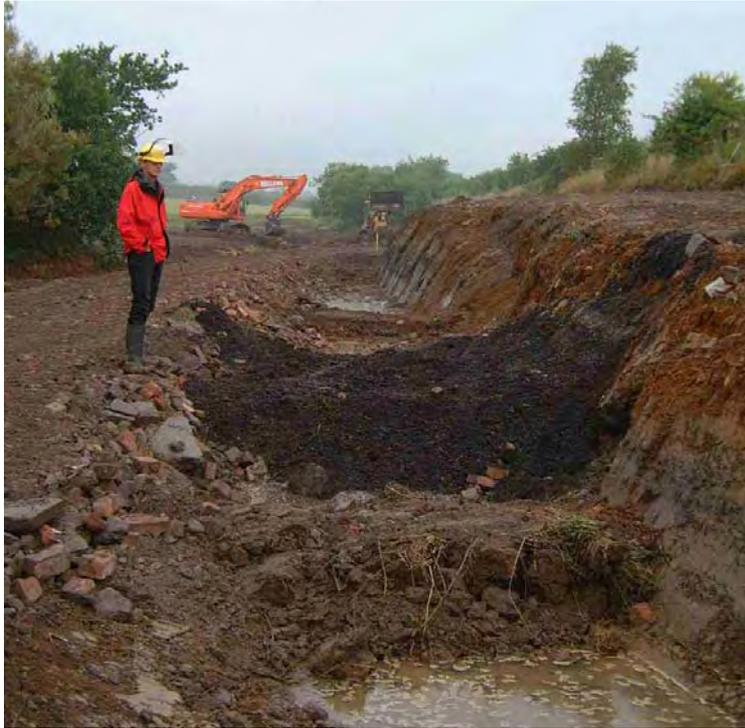
Figure 5.4. PRB construction: the first load of reactive media to be tipped into the trench, abutting the spoil on the right, and the demolition-rubble berm on the left (upon which Professor Andy Aplin is standing); the demolition rubble provides a permeable interface through which water can flow from the PRB into the settlement lagoons (being formed in the background).
