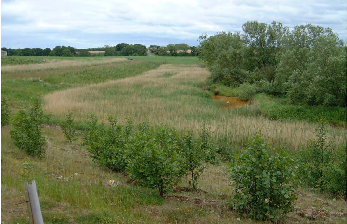
Figure 5.8. The pre-existing aerobic wetland at the site, which effects polishing treatment of the effluent from the settlement lagoons.
