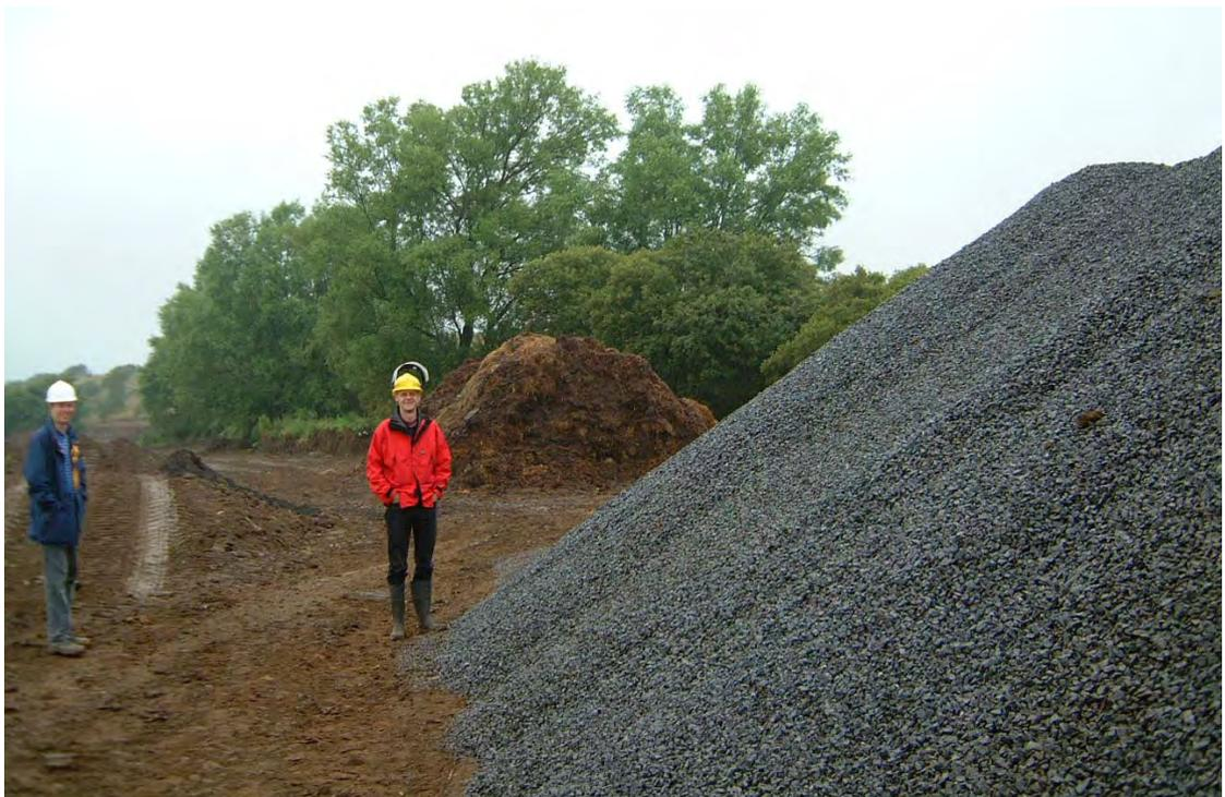
Figure 5.5. Stockpiles of manure and limestone, ready for mixing prior to placement in the PRB trench.
