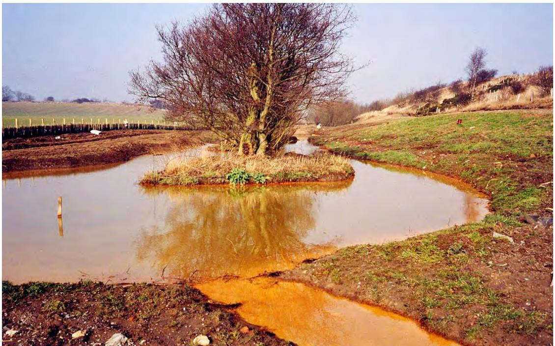
Figure 5.7. The settlement lagoons after completion and commissioning of the Shilbottle passive treatment system. The water flowing out of the lagoons is bright orange in colour due to the rapid hydrolysis and precipitation of iron in the presence of the alkalinity generated in the PRB.
