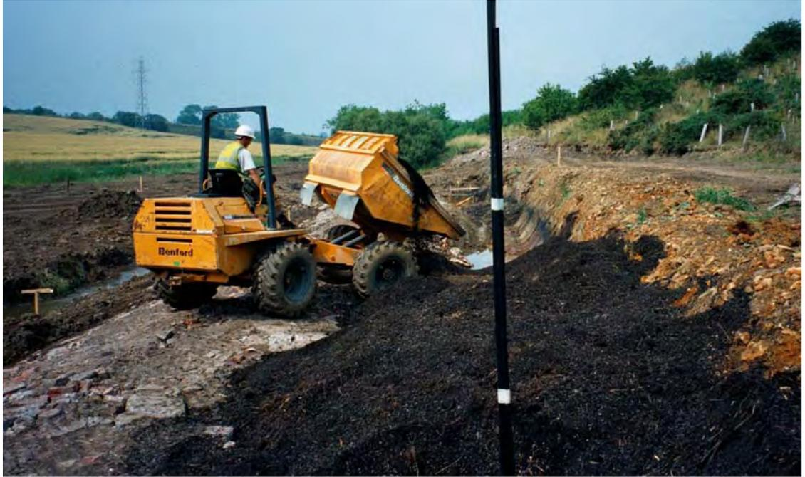
Figure 5.6. Mixed substrate being placed into the PRB trench. In the foreground a cluster of multi-level piezometers have been installed.
