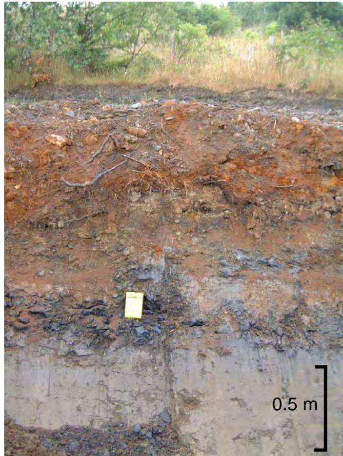
Figure 5.3. Excavation of the trench for the PRB underway, clearly indicating the contact between the (relatively permeable) oxidised colliery spoil (orange in colour) and the underlying, low-permeability boulder clay (dark grey in colour). The contact lies immediately below the notebook (there is minimal seepage of leachate at this particular point).
