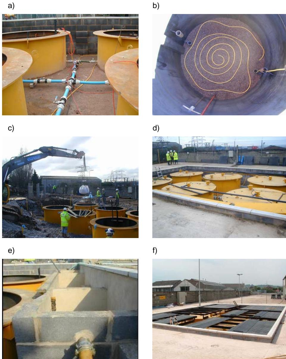
**Plate 6.2: a) connecting pipes, b) layout of the sparger system within a canister, c) filling the canisters with the reactive materials, d) vent pipework for collection of gases from the canisters, e) interceptor as a first stage prior to the entrance to the reactive canisters, and f) covering the canister system with a steel mesh grillage**
