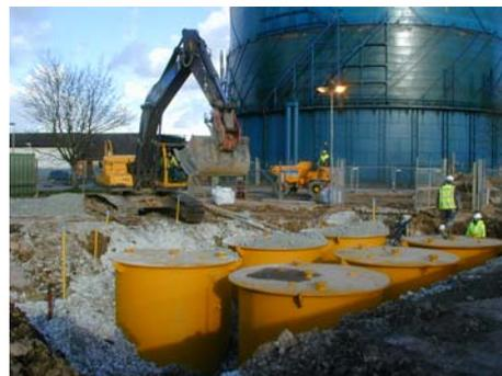
**Plate 6.1: Sequential images of the installation process of the SEREBAR: a) excavation of the cut-off trench, b) installation of a deep well downgradient of the reactive gate, c) lifting canisters into position, and d) backfilling space around canisters**
