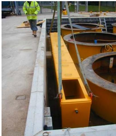
**Plate 7.1: Installation of the new interceptor**
