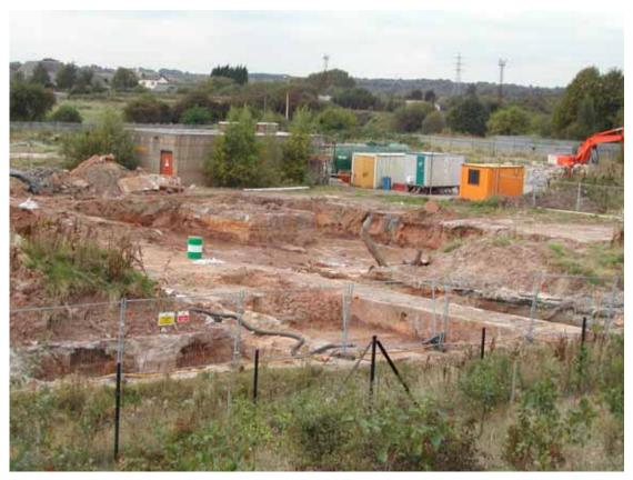
Plate 7.2: Excavation of Remediation Area.
