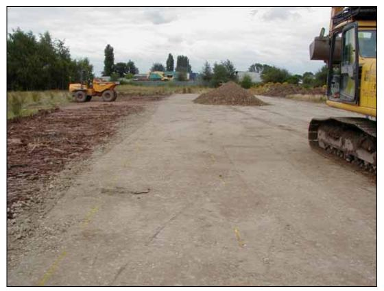
Plate 6.1: Construction of Treatment Bed Base.
