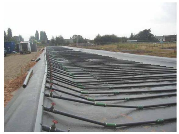
Plate 6.3: HDPE Liner and Vapour Extraction Pipe Array.
