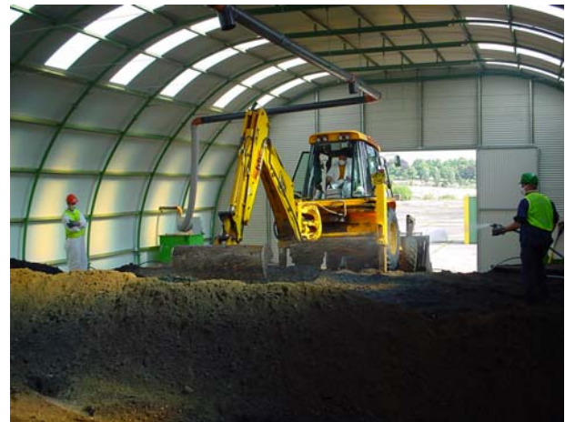
Spraying the biopile with water
