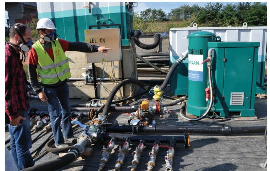
**Figure 2.** MPE vacuum extracGon pump.
