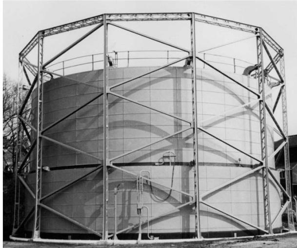
**Photograph 5.** A two-lift frame-guided gasholder with below-ground tank, using Cutler's patented system, Southern England. Source: IGEM PHI.
