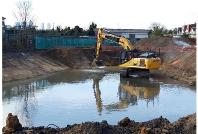
Figure 7: Photo showing that the depth of the dig was just beneath the groundwater level to reduce over-excavation.
