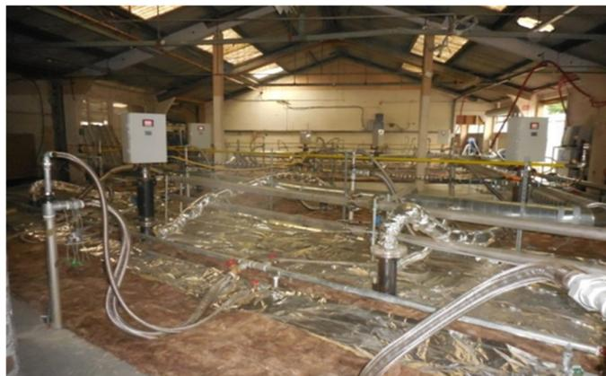
Figure 2: Heating and recovery well array.
