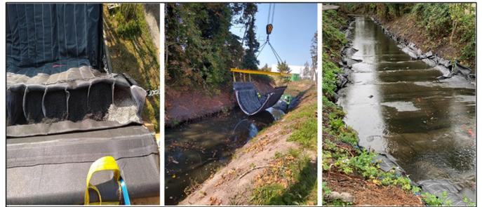
Figure 3: Construction of reactive mat in the Lieve.
