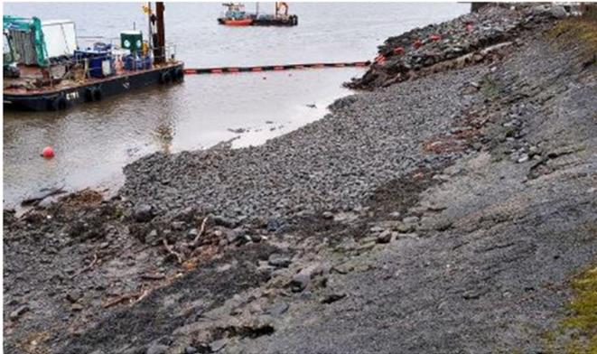
Figure 9: Area of filter stone placement.
