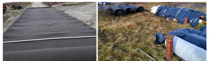
Figure 7: Rolled out RCM<sup>®</sup> and OBB geo-composite. Figure 8: Cut and rolled up segments or panels.
