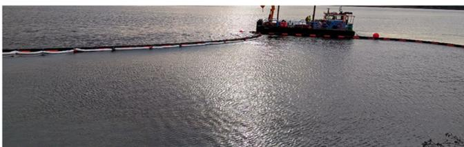
Figure 6: Floating containment and absorbents.
