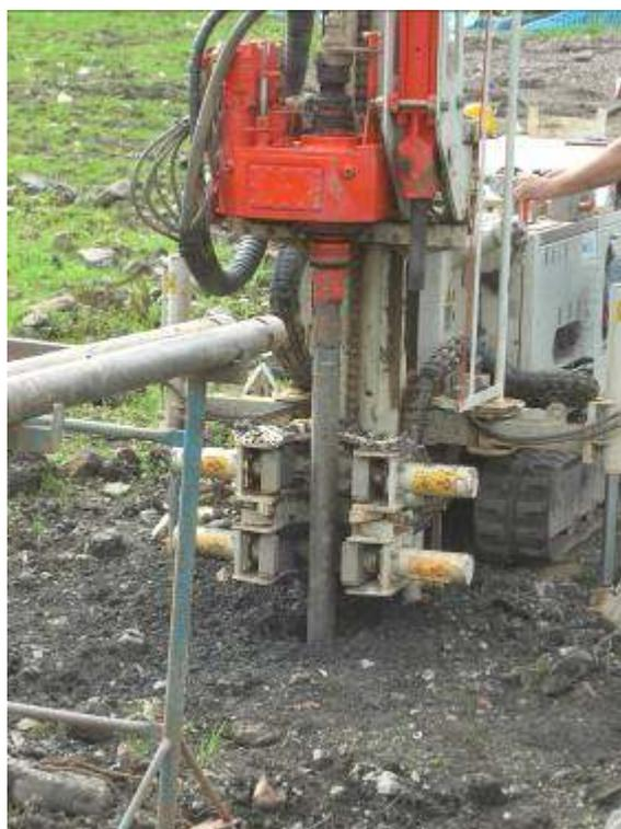
**Figure 4.65: Window corer used to extract the soil samples**
