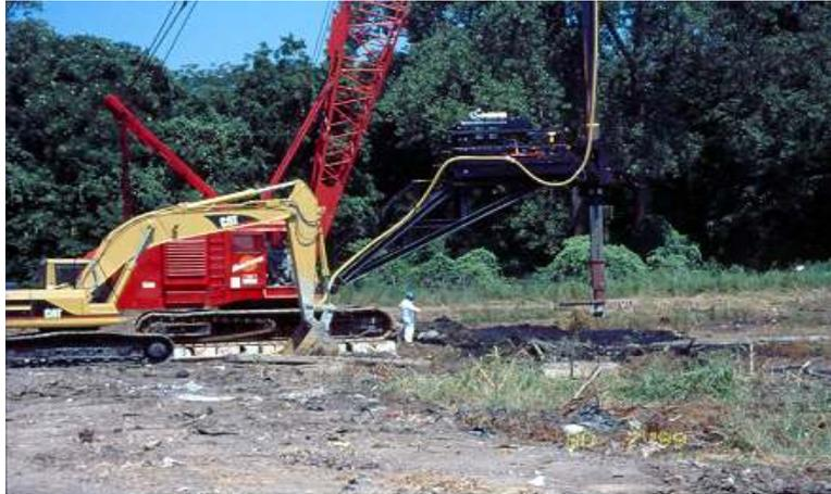
**Figure 4.42: Crane and Auger Assembly at South 8<sup>th</sup> Street**
