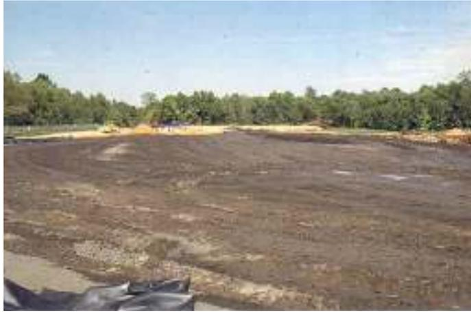
**Figure 4.15: Treated Soil Placement at American Creosote Site**
