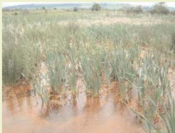
Figure 9: St Helen Auckland - an aerobic reed-bed treating net-alkaline mine water.
