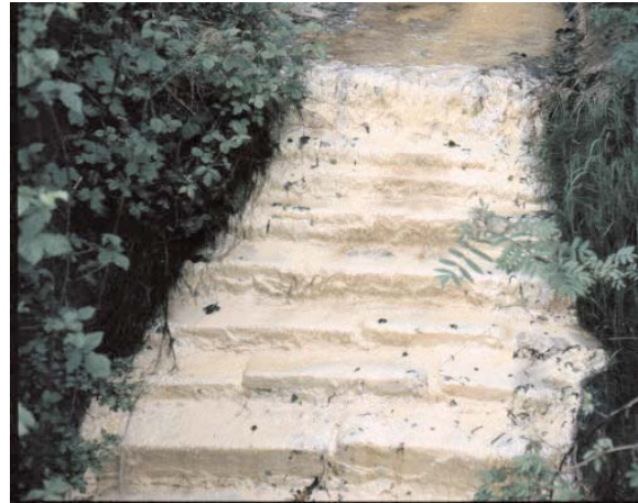
Figure 3: Aluminium hydroxide deposition from one of the acidic discharges at Bowden Close, prior to remediation.
