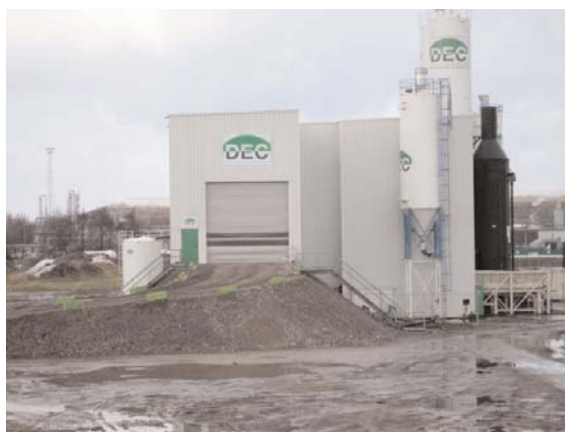
Figure 11: DEC solidification plant near Reime, Belgium.
