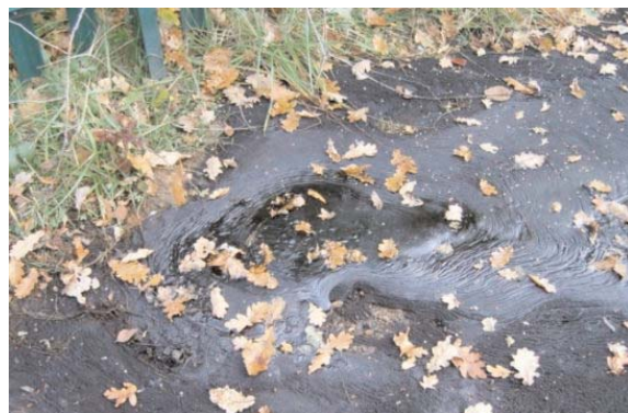
Figure 4: Tar that has bled through the subsurface and is slowly flowing over grass.
