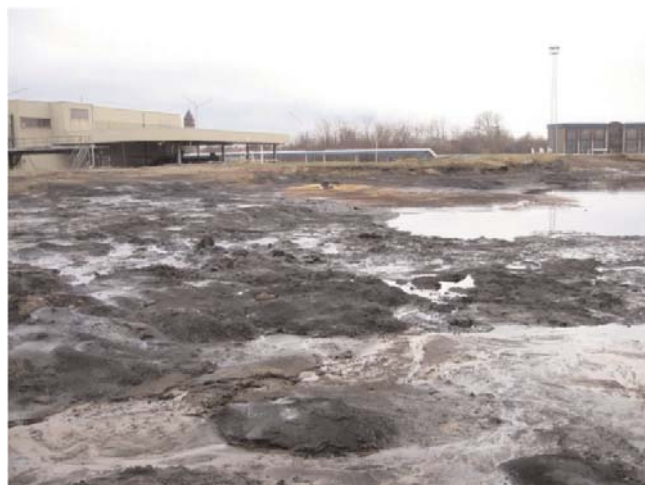
Figure 1: Acid tar lagoon, Rieme, Belgium.
