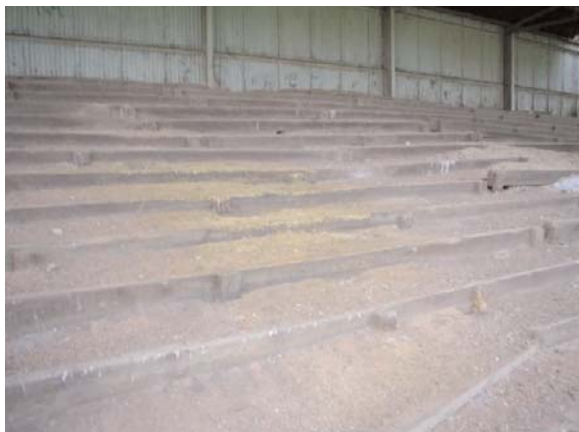
Fig.2: Visible chromium contamination from COPR in the stands at a stadium in Shawfield.
