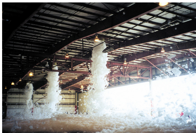
Figure 3. Foam generators used to dispense high-expansion foams (Image courtesy of National Foam).
