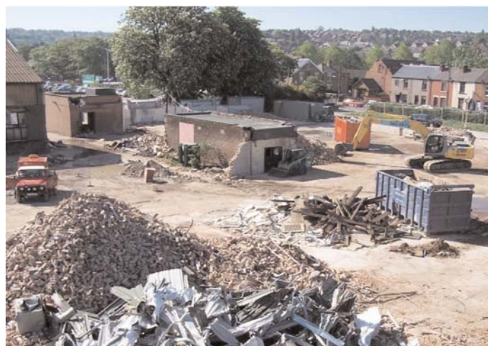
Figure 4: Demolition in progress
