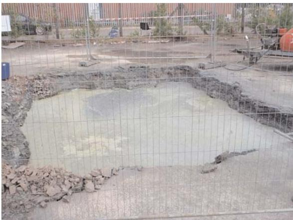
Figure 10: Settlement of ground in area of plot following completion of soil mixing trial
