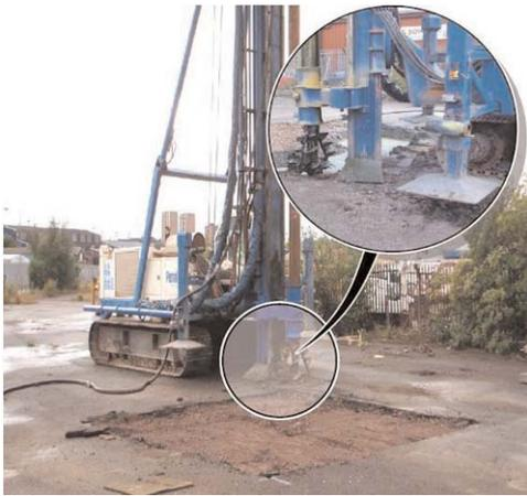
Figure 9: Rig used for soil mixing trial
