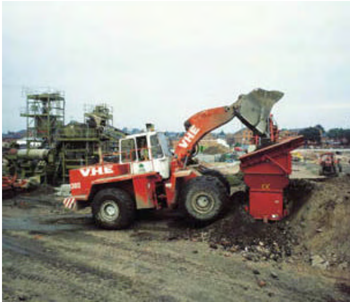
Plate 1: Pre-screening of excavated material for feed to soil washing plant.
