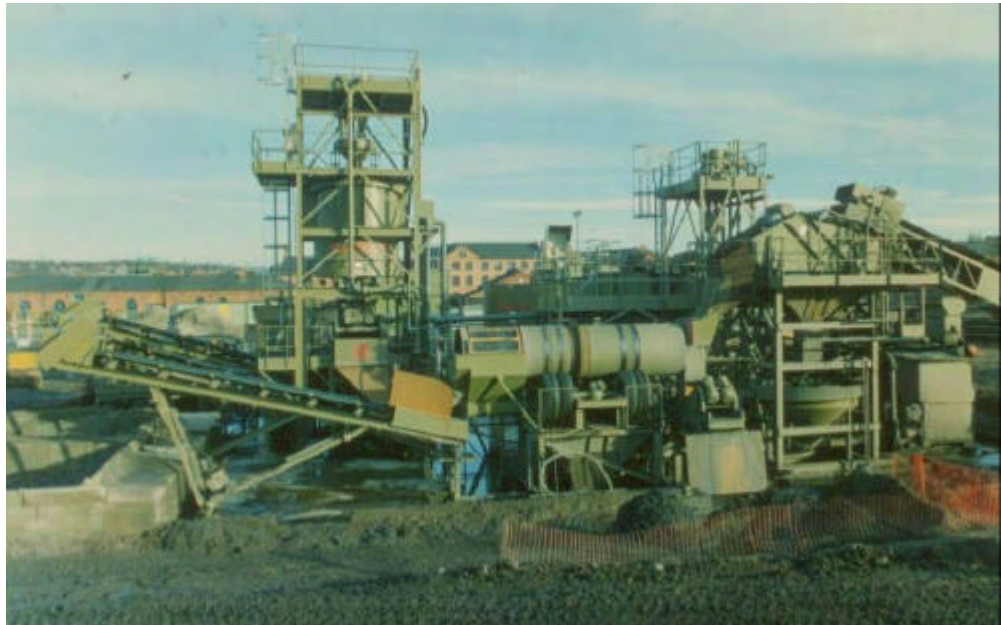
Plate 7.1: Soil washing plant.
