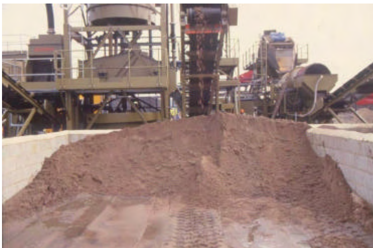
Plate 3: Clean sand output from soil washing plant.
