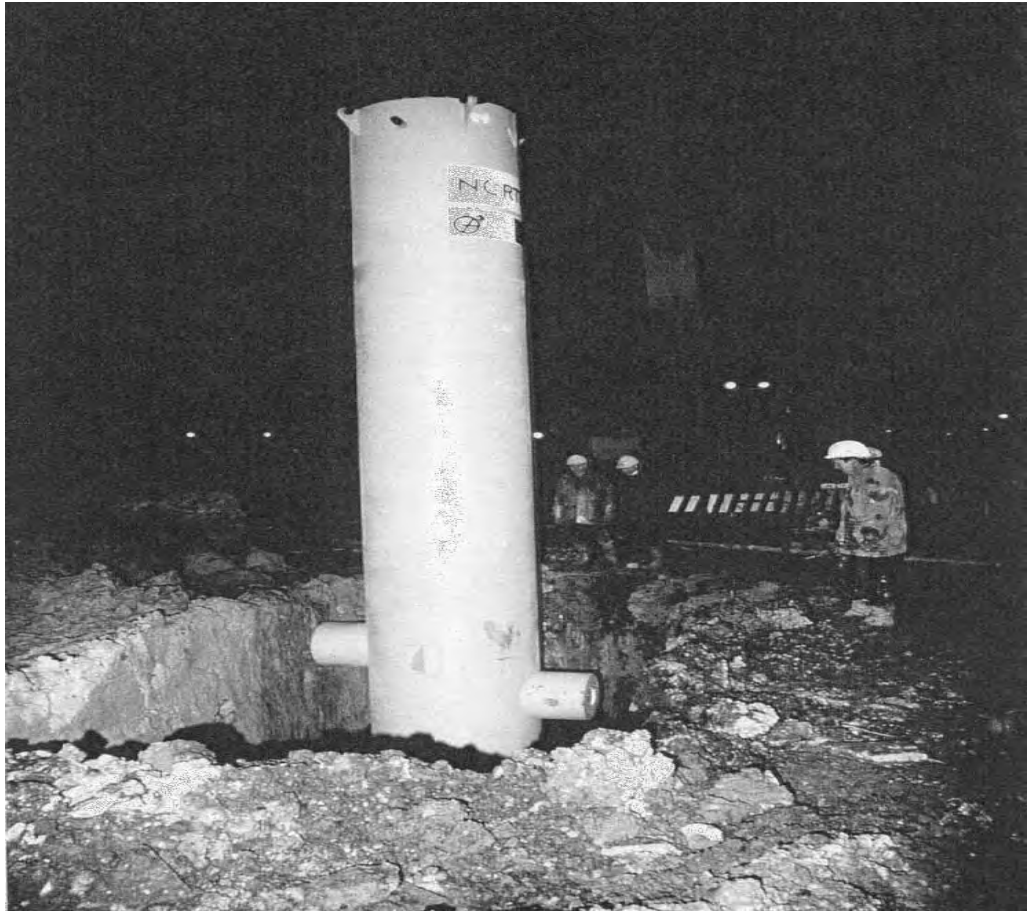
Plate 6.4: Reaction vessel aligned for installation
