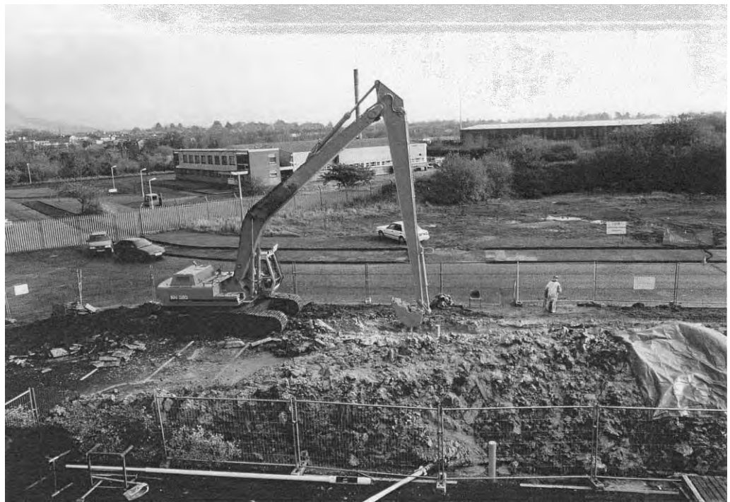
Plate 6.1: Modified backhoe excavating trench
