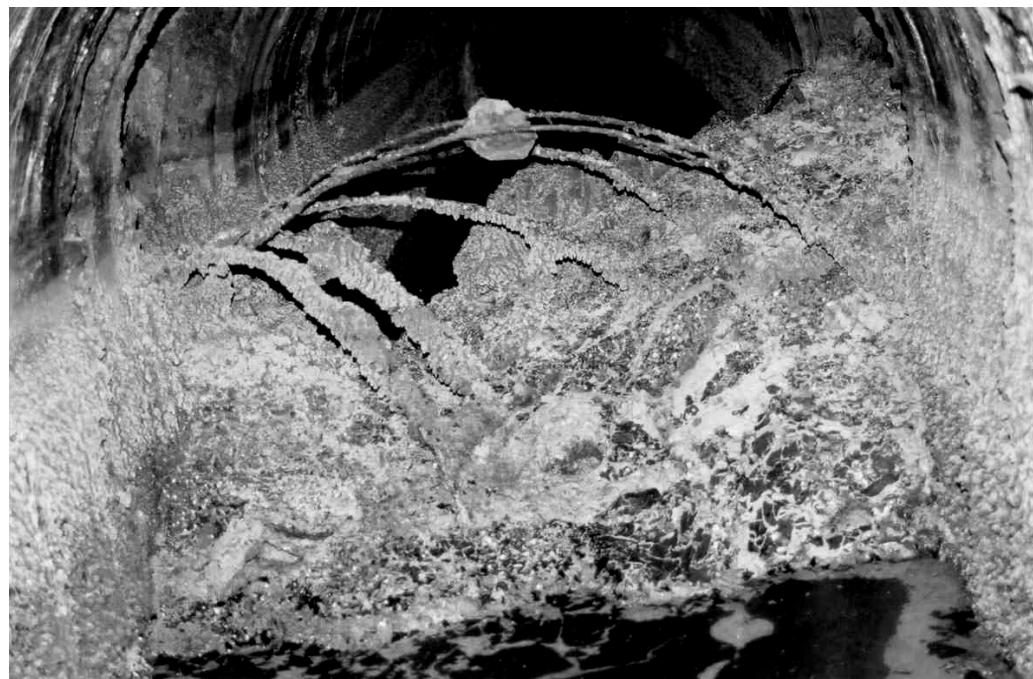
Figure 2.2: View inside Harvey Drift (representing Discharge No 1 at Bowden Close) showing roof collapse into workings.
