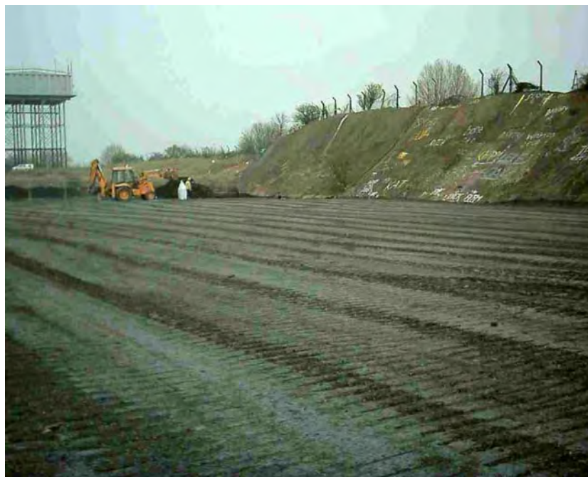
Plate 7.1: Biopile base following completion
