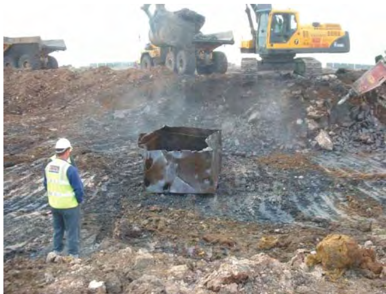
Plate 6.2: Supervision of the excavation process
