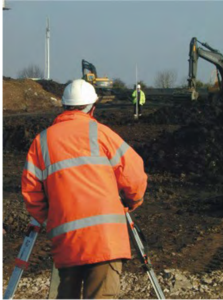
Plate 6.1: Surveying of the sampling grid
