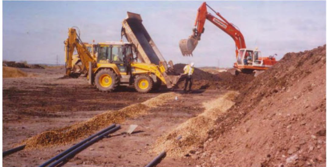
Plate 7.2: Biopile formation works
