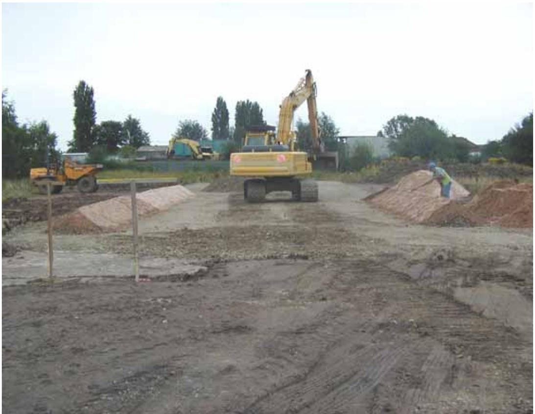
Plate 6.2: Construction of Treatment Bed Base and Containment Bunds.
