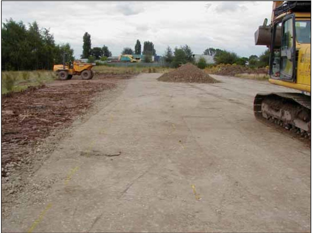
Plate 6.1: Construction of Treatment Bed Base.
