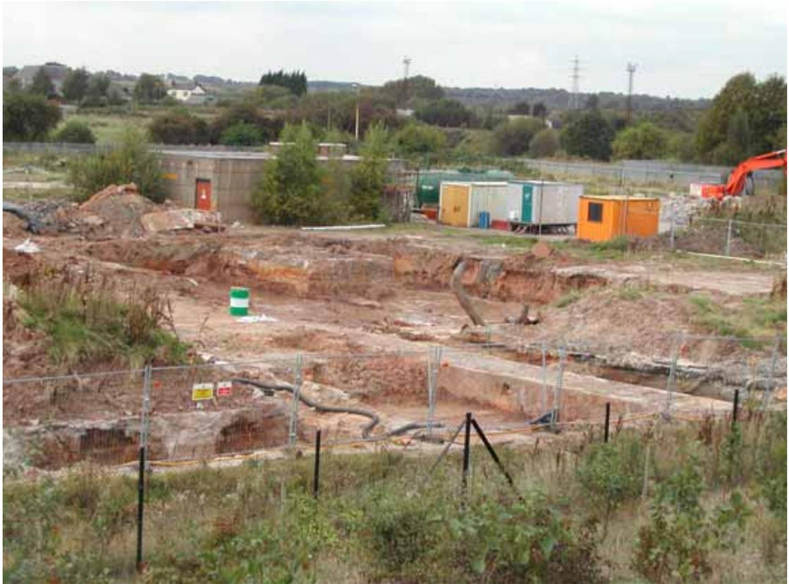
Plate 7.2: Excavation of Remediation Area.
