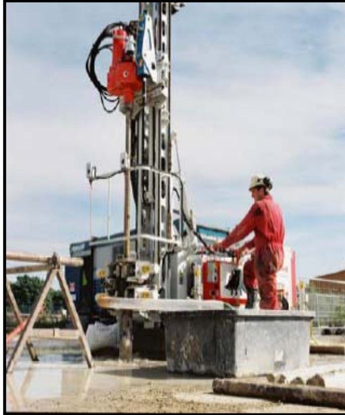
Plate 3.3: Rotary coring of characterisation boreholes
