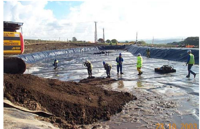
Earthworks for the treatment system at Bowden Close.
