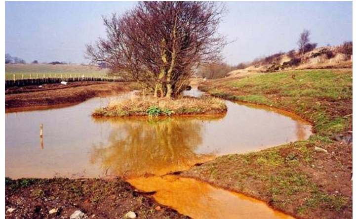
The settlement lagoons after completion and commissioning of the Shilbottle passive treatment system. The water flowing out of the lagoons is bright orange in colour due to the rapid hydrolysis and precipitation of iron in the presence of the alkalinity generated in the PRB.
