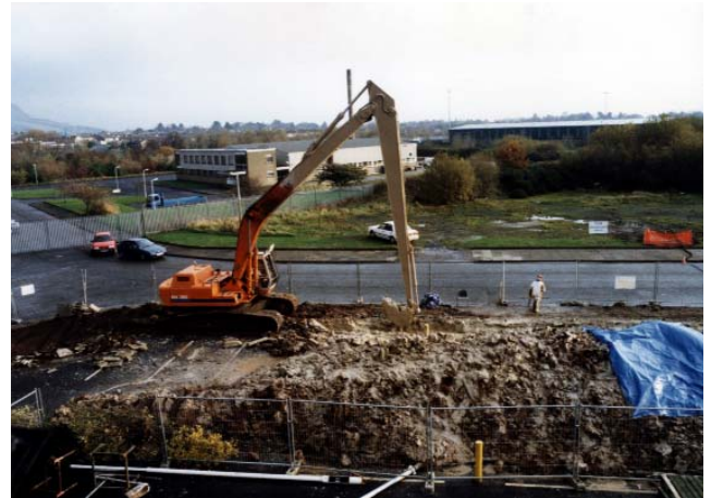
Modified backhoe excavating trench
