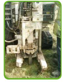
Figure 3.2: Drilling of boreholes (part of the Site Investigation)
