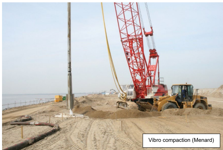
Figure 3.17: Vibro compaction
