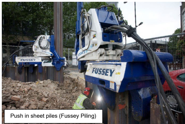
Figure 3.23: Push or press in sheet piles
