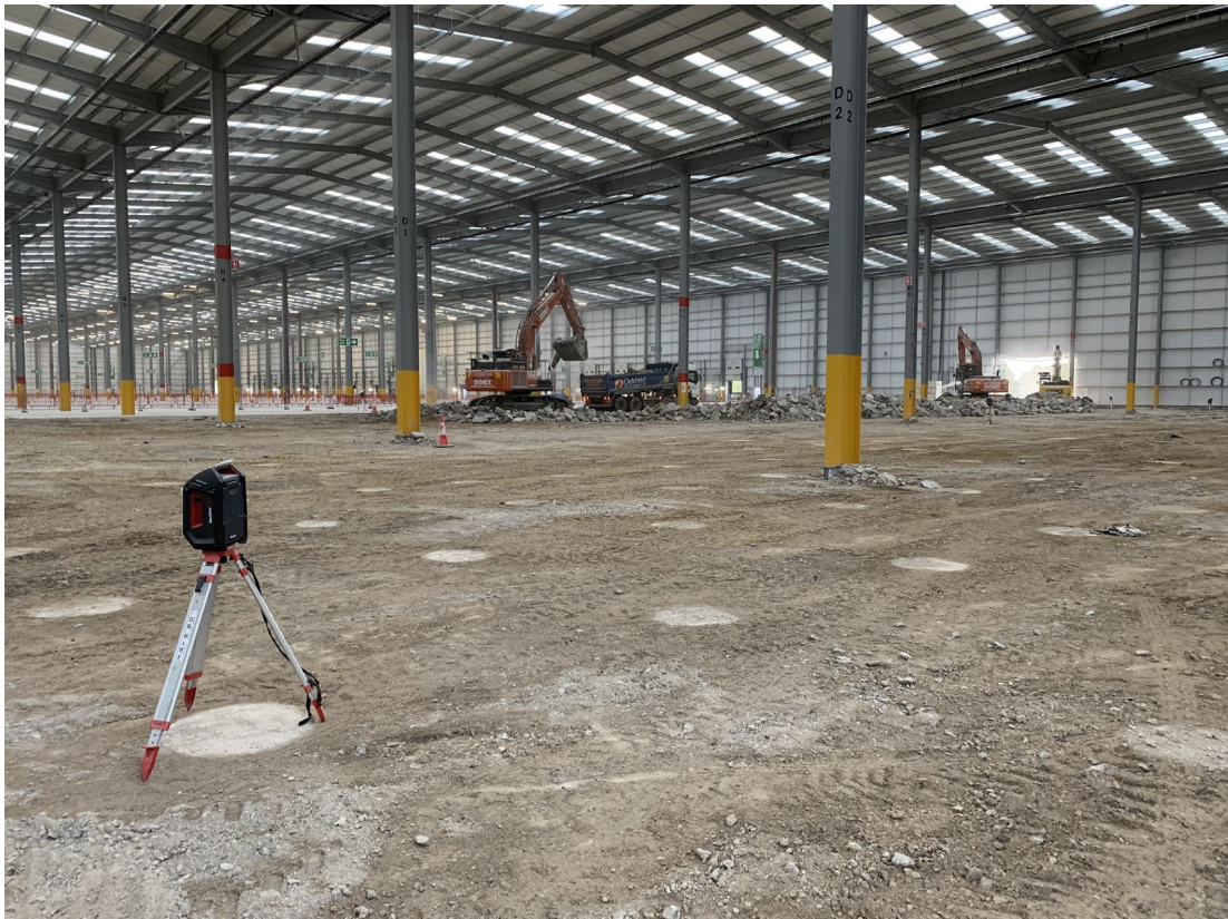
Figure A2.17: Area monitoring for flammable gas above exposed piled foundations
