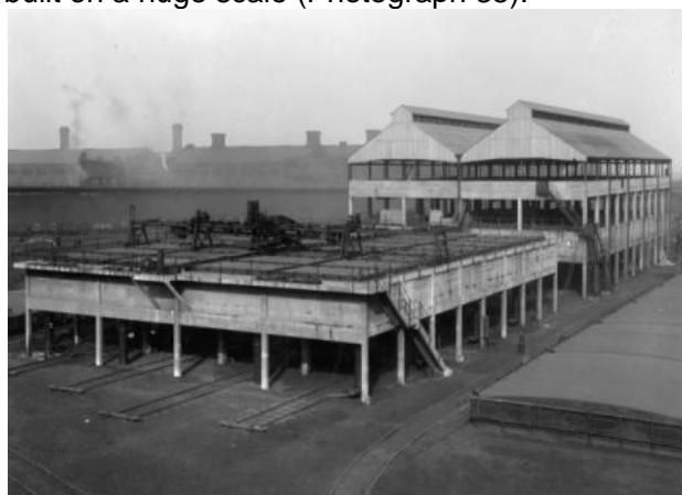
Photograph 35. A large purifier house.
