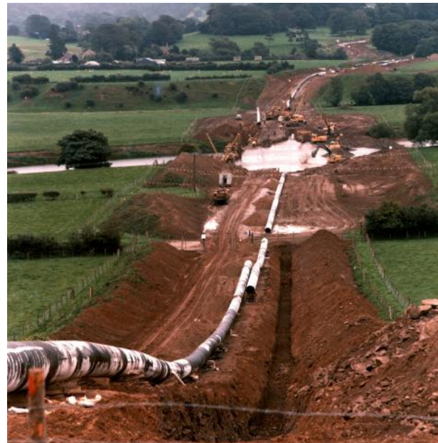
Photograph 12. Building the National Transmission System.
