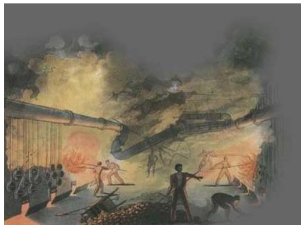
Figure 4. An early painting depicting conditions within Brick Lane gasworks.
