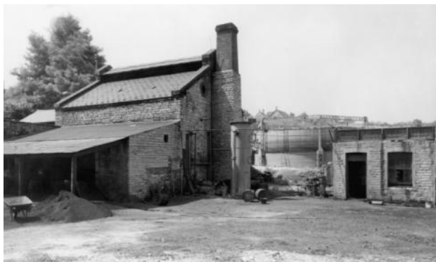
Photograph 15. A typical village gasworks in Somerton, Somerset. The main building is the retort house, the gasholder can be seen behind.
