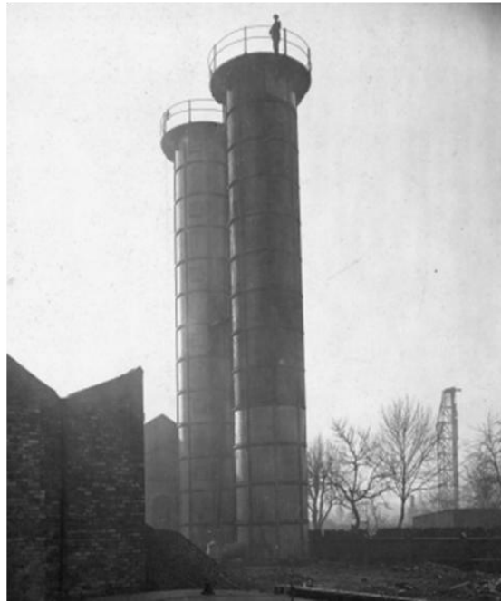
Photograph 31. Two tower scrubbers.
