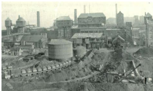
Photograph 54. The sulphuric acid plant at the Beckton gasworks.
