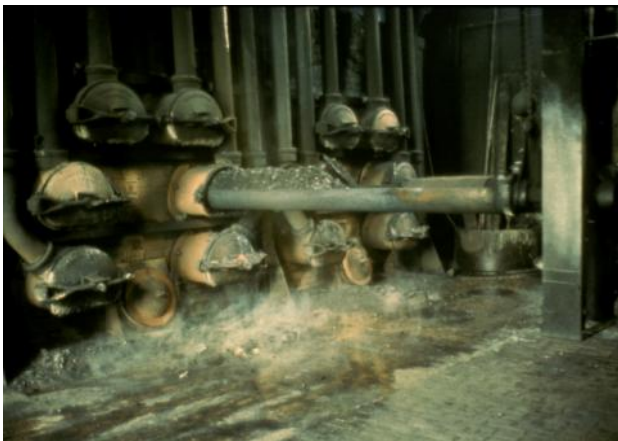
Photograph 21. Loading a retort with a mechanical charger.
