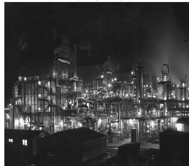
Photograph 58. Reforming plant at Ambergate, Derbyshire.
