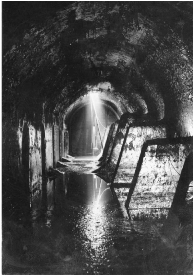
Photograph 43. Interior of a tar tank at the former gasworks, Sydenham.
