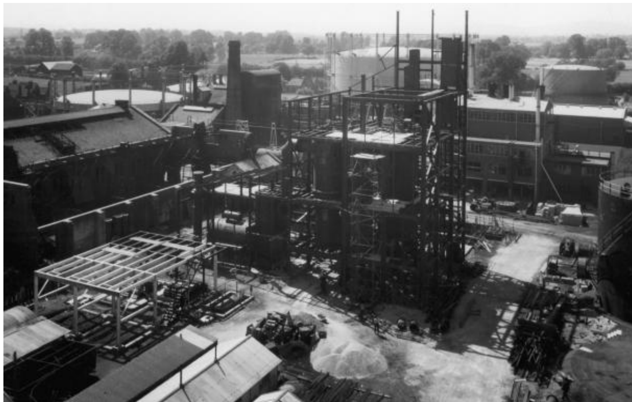
Photograph 57. The Hempsted gasworks Gloucester, where a range of oil gasification processes were constructed, including the Hall, Jones and Gas Integrale processes.
