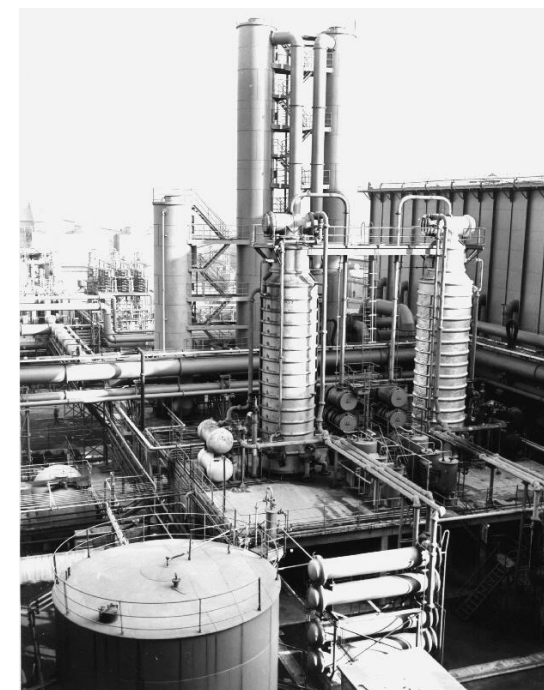
Photograph 47. Large benzole plant at the former Carr House gasworks in Rotherham.
