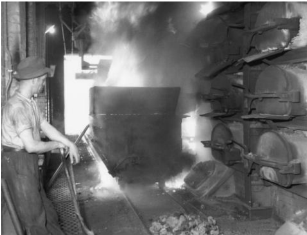
Photograph 20. Unloading a through-ended retort mechanically.
