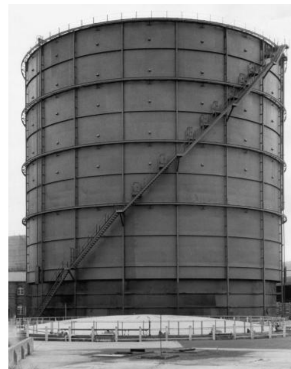
Photograph 40. Waterless gasholder of the Wiggins design.
