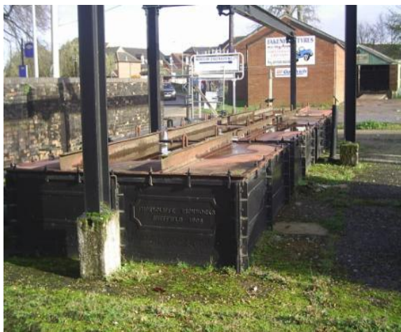
Photograph 34. An example of box purifiers at the Fakenham Gas Museum, Norfolk.
