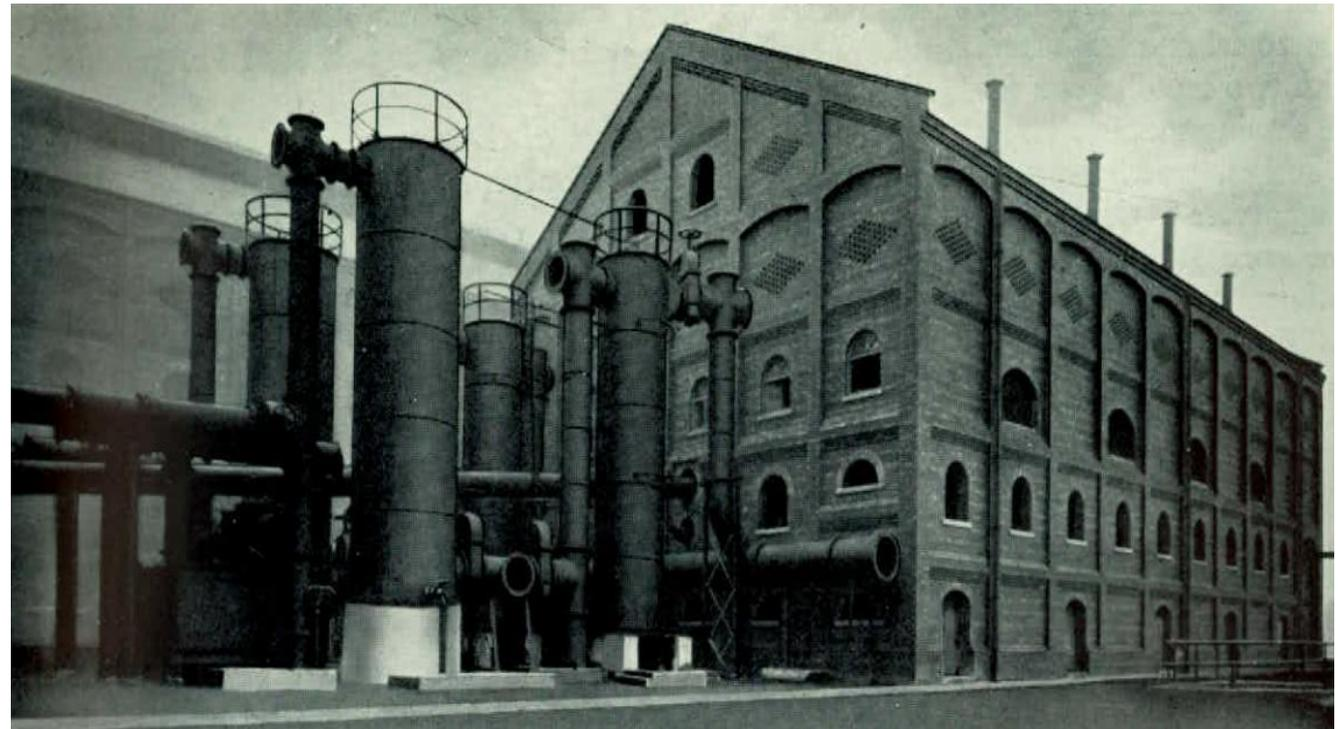
**Photograph 3. The Trefois producer house, built by Drakes at the Partington Gasworks, Manchester, which supplied producer gas to the retorts. The ancillary washers and scrubbers can be seen outside the building. Source: National Grid Gas Archive.**
