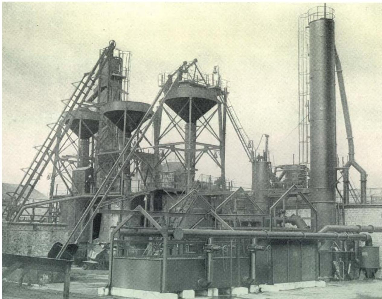
**Photograph 8. A producer gas plant with cooling and purifying plant for gasification of bituminous coal. Source: National Grid Gas Archive.**
