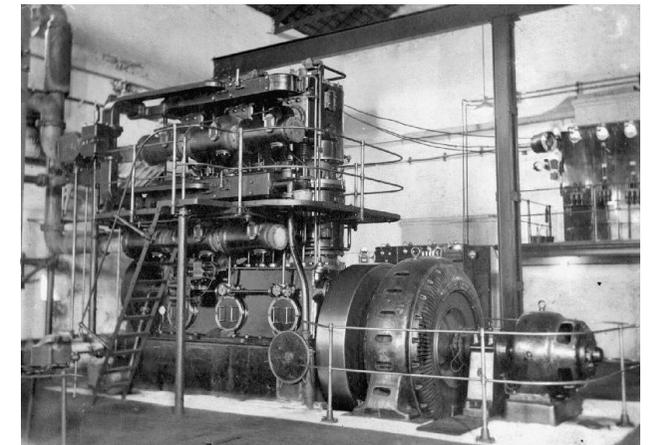
**Photograph 5. Gas engine powering an electrical generator at a colliery powerhouse, 1914. Source: National Grid Gas Archive.**
