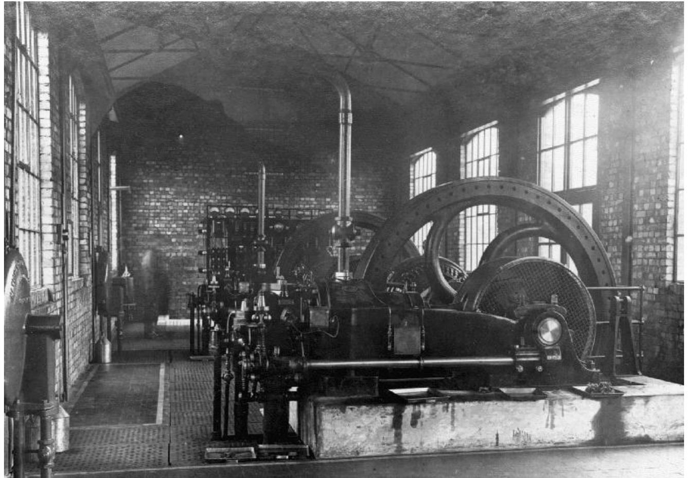
**Photograph 2. Two gas engines installed at the former Wandsworth power house. Source: National Grid Gas Archive.**
