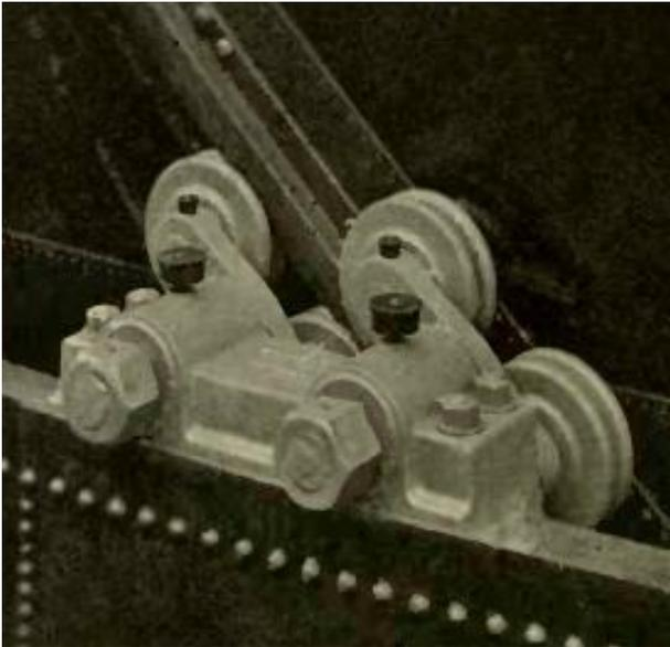
**Photograph 8. Multiple Roller Carriage which guides the upwards and downwards movement of the spiral gasholder. From *Modern Gasworks Practice* by Alwyn Meade.**
