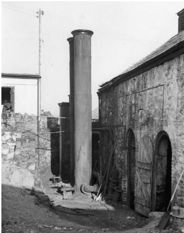
**Photograph 23. A set of two atmospheric condensers, Gunnislake gasworks, Cornwall.**
