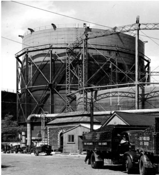
**Photograph 6. A gasholder fitted with a flying lift.**
