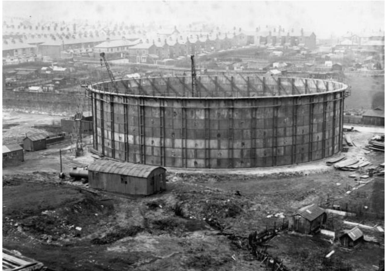
Photograph 15. Construction of an above-ground steel tank.
