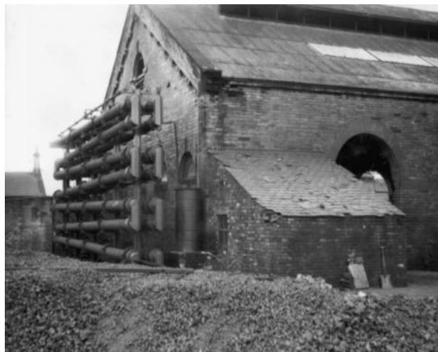
**Photograph 24. A horizontal atmospheric condenser.**
