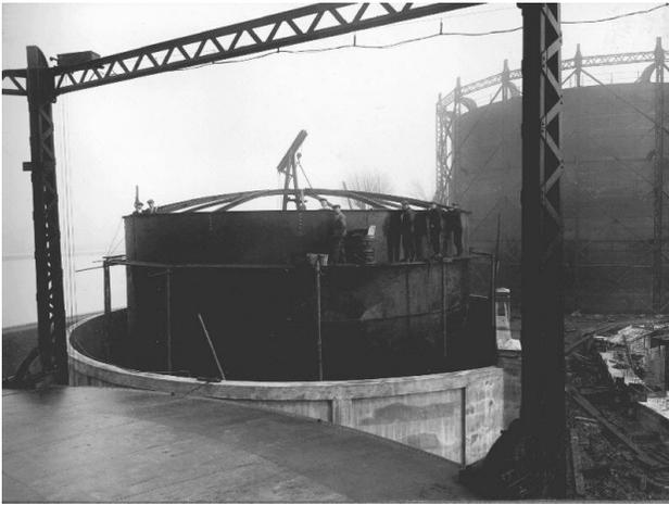
**Photograph 11. Construction of a traditional above-ground oil storage tank at Brentford Gasworks in 1929, showing the perimeter wall protecting the tank and the construction of the tank roof and walls. Source: National Grid Gas Archive.**
