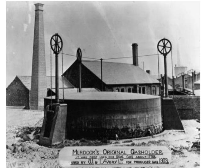
**Photograph 4. Murdoch's original circular gasholder at the Soho works.**
