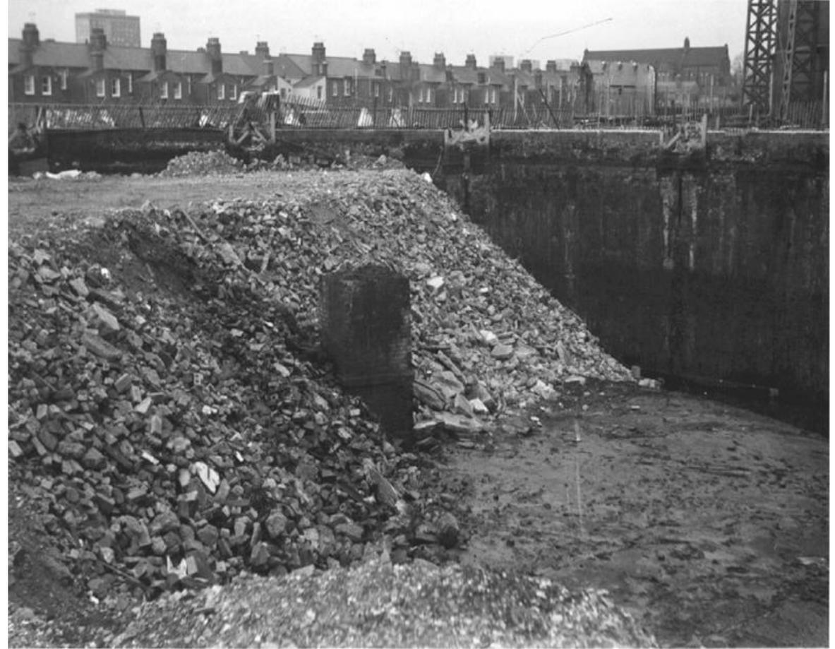
Photograph 14. The decommissioning of a gasholder at Croydon in the 1970s. Removal of the guide-frame standards (left) and the partially infilled gasholder tank (right).
