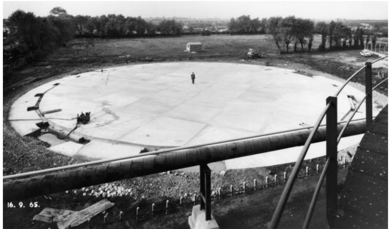
**Photograph 12.** Concrete foundation slab of an above-ground gasholder.
