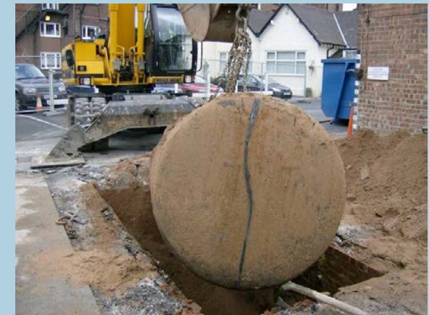
FIGURE 17 Empty tank lifted
