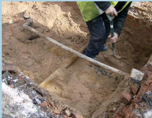
FIGURE 15 Bedding material removed by hand
