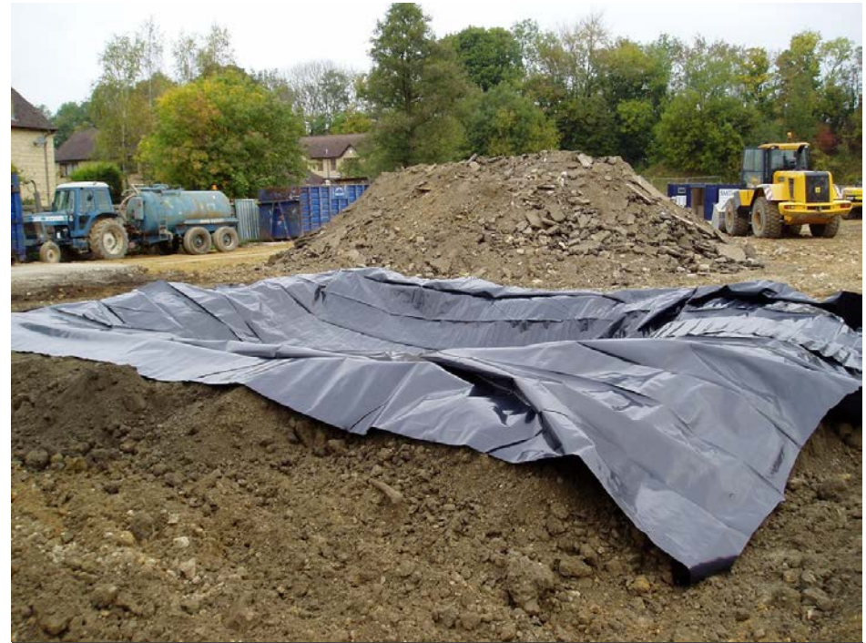
FIGURE 8 Temporary contaminated groundwater lagoon
