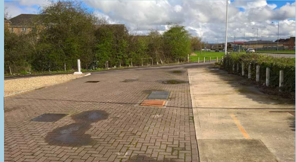
FIGURE 11 Inspection chambers at disused forecourt
