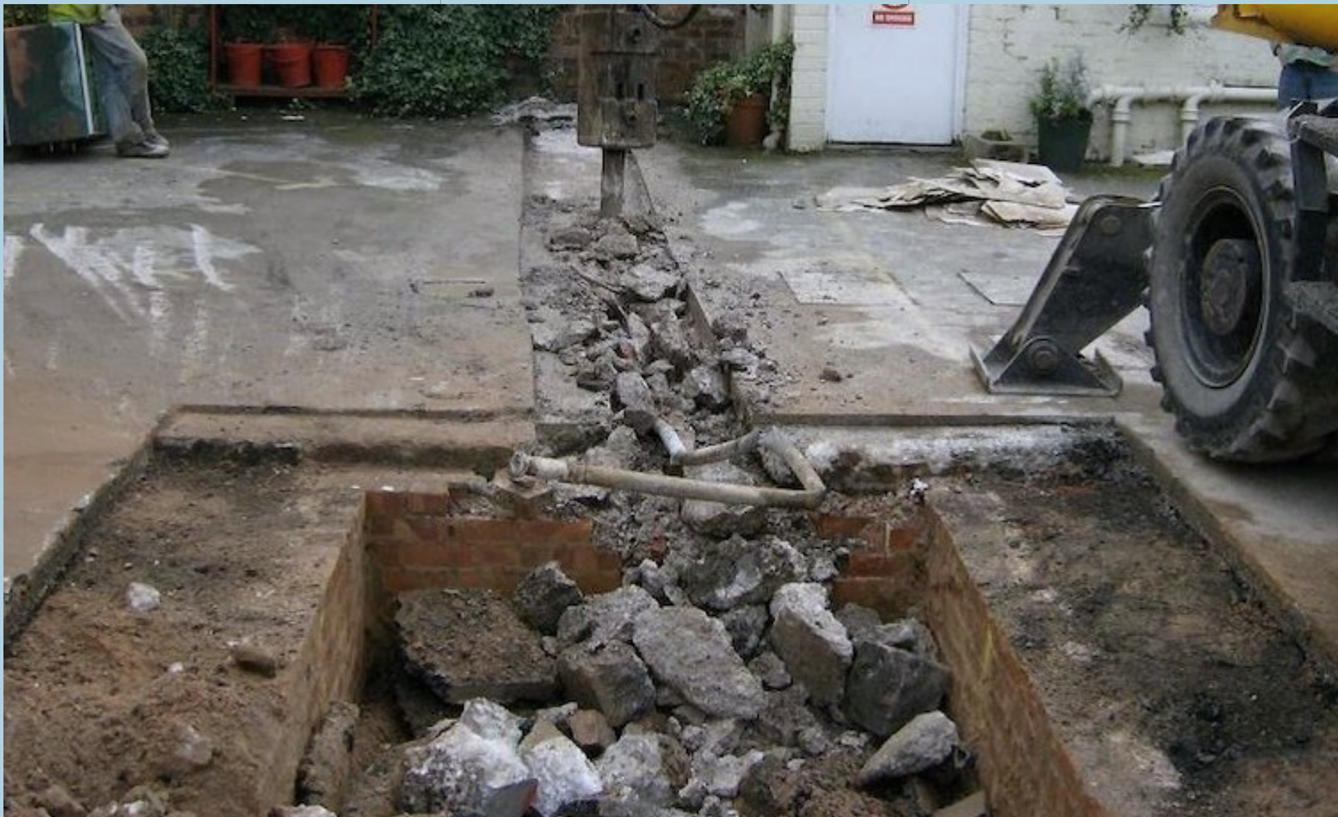
FIGURE 18 Pipework removed and tank housing area backfilled
