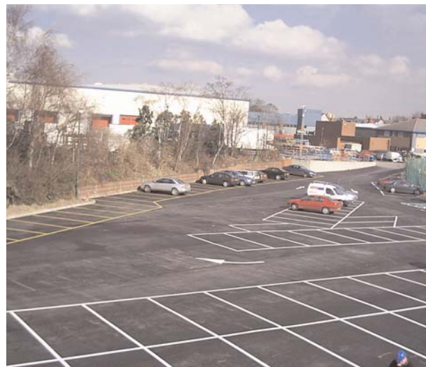
South Car Park post remediation 2005
