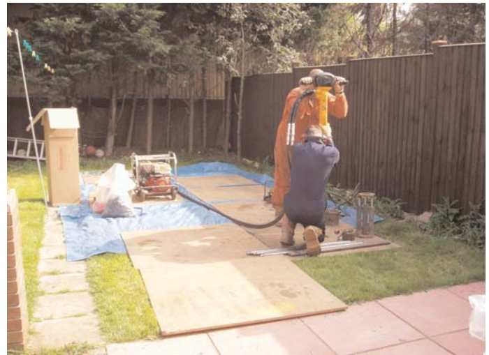
Care was taken to minimise damage to gardens
