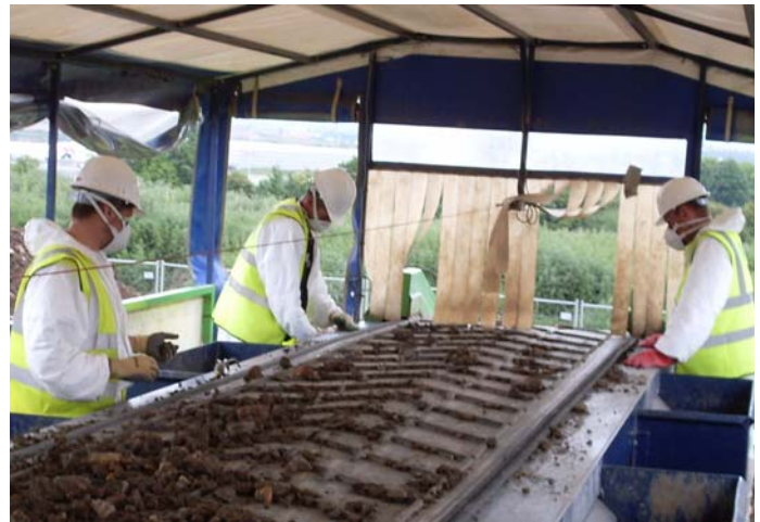
Figure 4. Asbestos picking station at the Donor site
