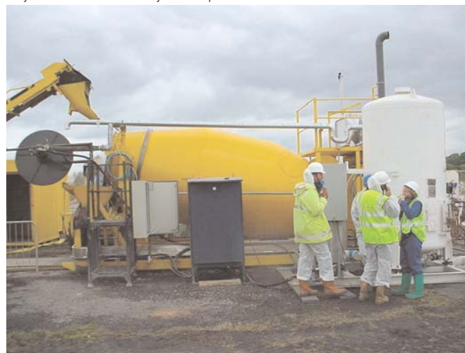
Figure 3: Carbonation chamber (centre) and carbon dioxide storage cylinder (right).
