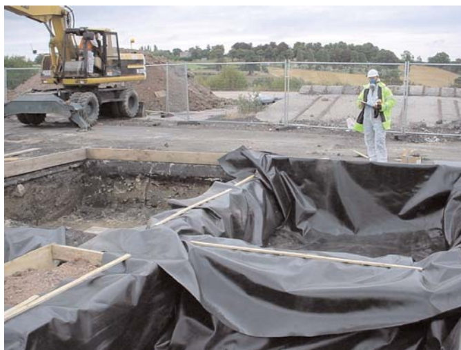
Figure 2: Treatment cells before being filled with treated material.
