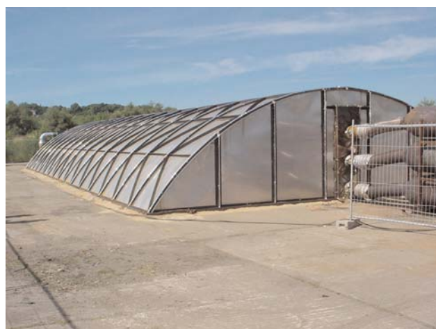
Figure 1: The completed thermal treatment cell from the burner end.
