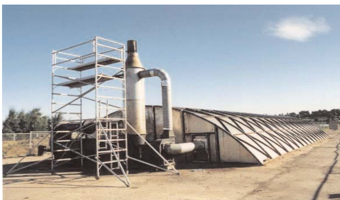
Figure 5: Completed Treatment Cell 2, from the thermal oxidiser end.
