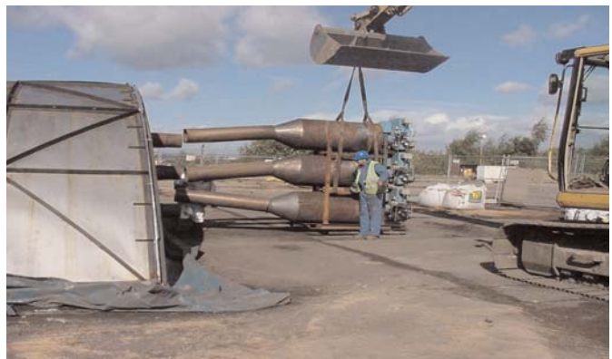
Figure 4: Fitting the burners.
