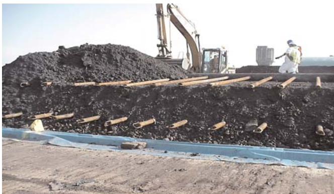
Figure 2: Building up the layers in Cell 1.
