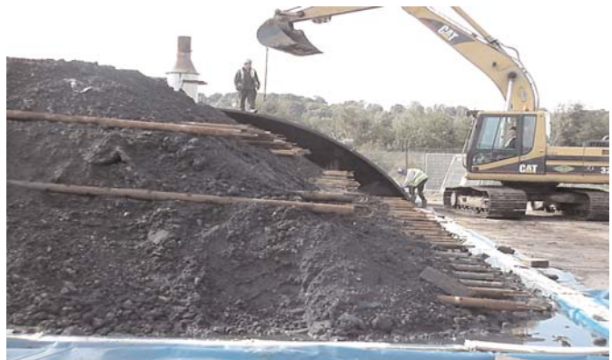
Figure 3: Moving the stainless steel panels into position.
