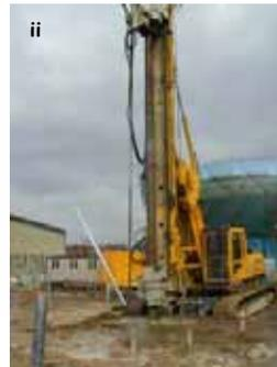
Schematic diagram of drilling, treatment cell preparation, pylon installation, *in situ* nutrient addition and sampling/monitoring in South West England (i). Picture of soil mixing rig at treatment cell 6 with U100 pipes before recovery for *ex situ* monitoring of soil columns in microcosms (ii).
