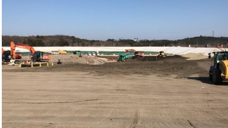
Interim storage facility
