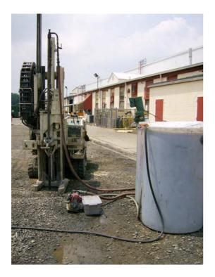
Figure 2 - Direct Injection of Iron NPs in the Field at the Trenton Facility, New Jersey (Photo courtesy of Geosyntec Consultants)
