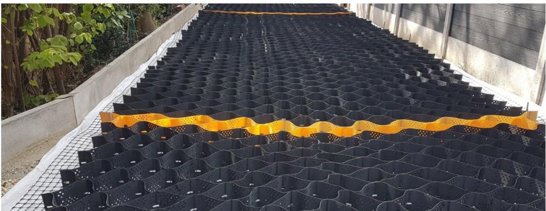
**Figure 3:** A geocell sheet laid in place prior to being filled with stone (image courtesy of Core LP)
