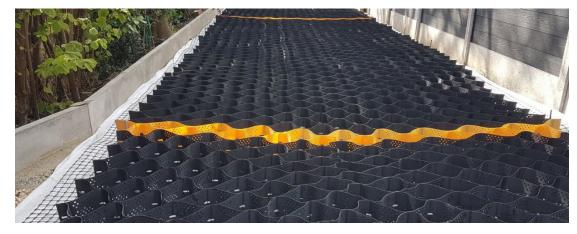
Figure 3: A geocell sheet laid in place prior to being filled with stone (image courtesy of Core LP)
