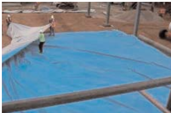
Figure 3. Installation of a horizontal root barrier membrane.
