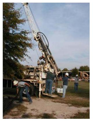
Figure 4.54: Drilling rig at the Columbus MGP
