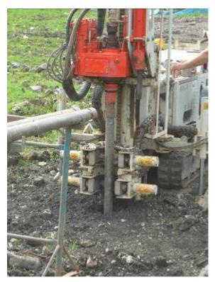
Figure 4.65: Window corer used to extract the soil samples
