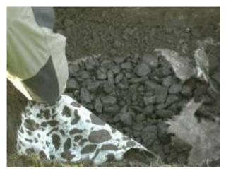
Figure 4.56: Layering on site, above the stabilised monolith
