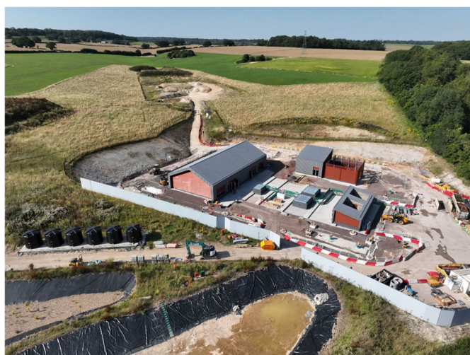
Figure 5: Chalfont St Giles Vent Shaft under construction in 2024.
