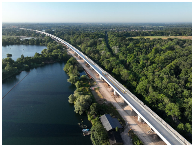
Figure 3: Colne Valley Viaduct (2024).
